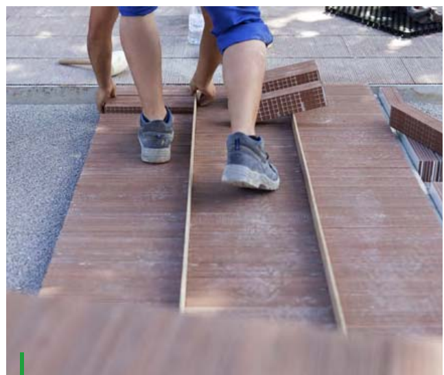
Permeable ceramic cobble installation
